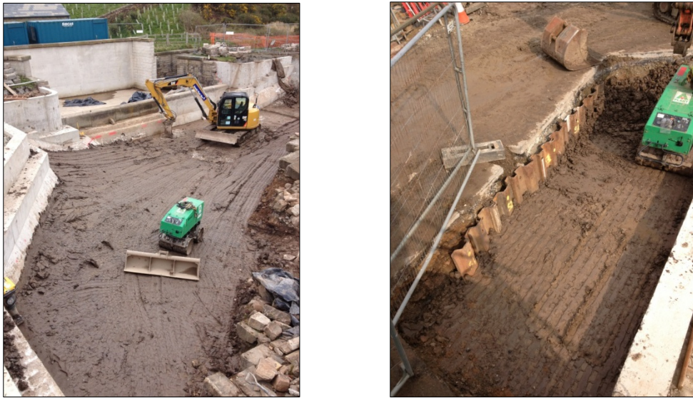
Figure 7. Clay blanket and core reinstatement
