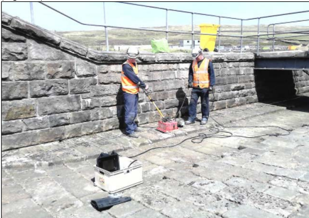
Figure 2. Application of GPR Survey
