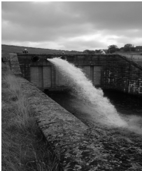
Figure 4: Valve test during commissioning at Pitsford
