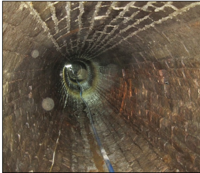
Figure 9. Drawoff Upstream Culvert After Cleaning
