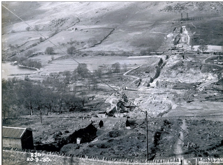
Figure 2: Initial excavations for foundations underway (1935)
