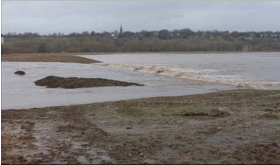
Figure 5. Inlet Spillway, Boxing Day Floods 2015
