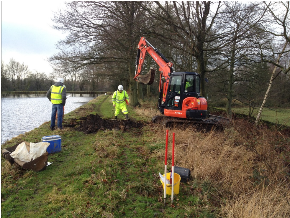
Figure 3 – Site Investigation trial hole at Swiss Lake
