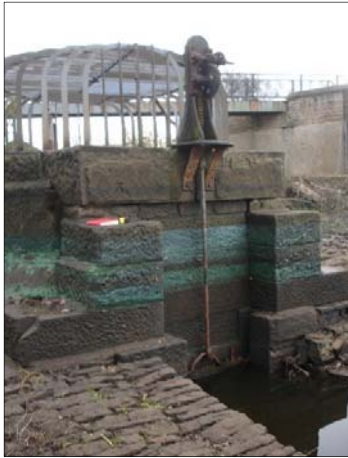
Figure 4. Existing Outlet Penstock.
