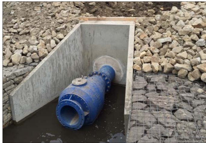
Figure 3: Wessenden Old IR Siphon inlet arrangement during construction
