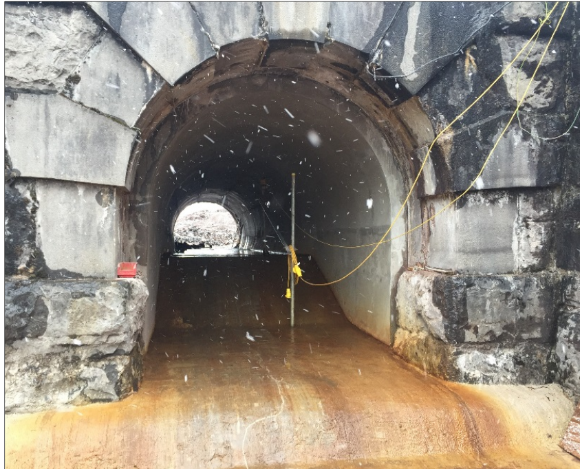
Figure 6. Construction stage: tunnel lining from downstream end
