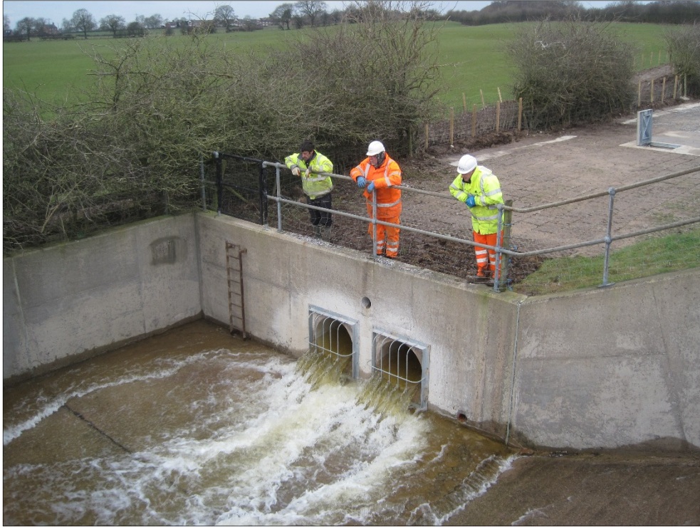
Figure 8. Siphon test, discharge into service spillway system
