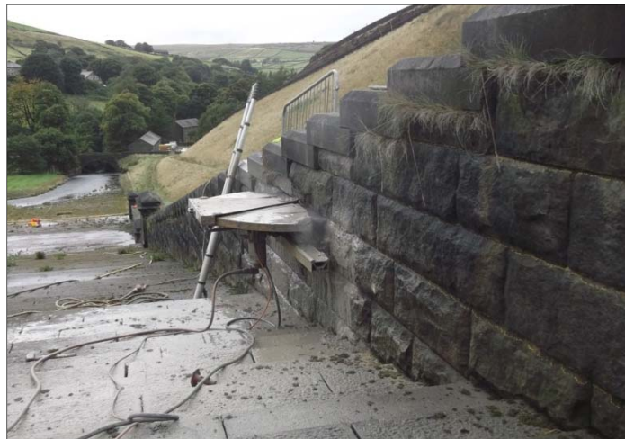
Figure 4 - Photograph of RHS spillway wall dismantling
