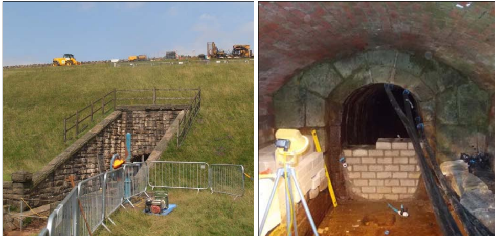
(a) Permeation grouting from crest (b) Tunnel infilling operations
