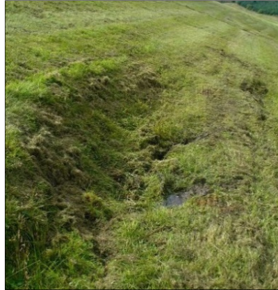
Figure 2. Wet patch on face
