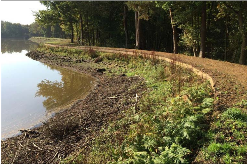
Figure 9 – Emperor Lake embankment raising works completed
