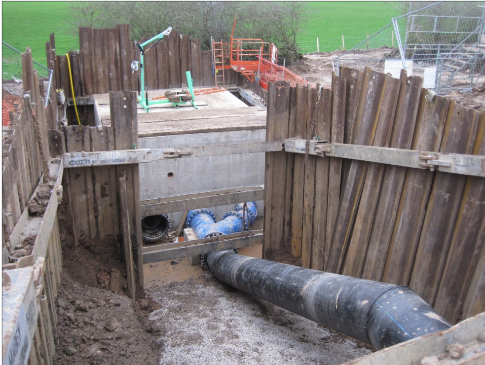
Figure 5. Pipework being laid under the downstream shoulder
