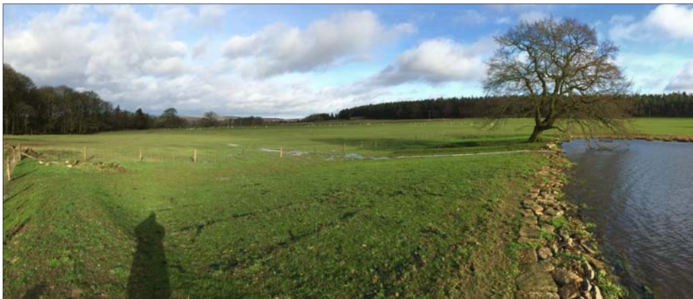
Figure 11 – Completed Spillway at Mud Pond
