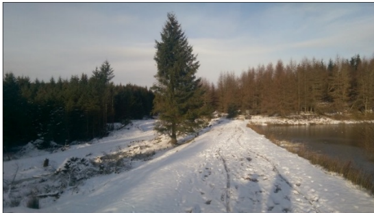
Figure 5: Greenlands No.1 dam crest
