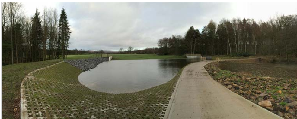
Figure 12 – Completed Causeway and Weir Structure at Emperor Lake
