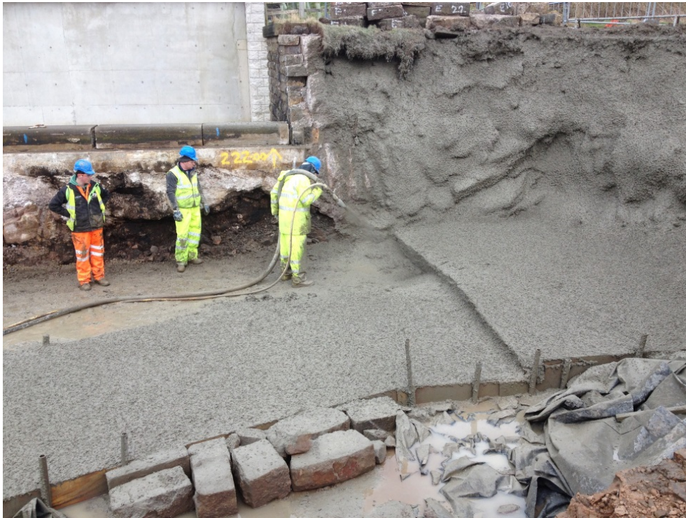
Figure 6: Fibre reinforced concrete installation
