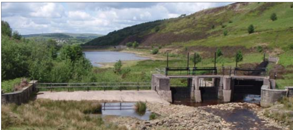
Figure 1. The former reservoir from the Inlet structure, looking west.
