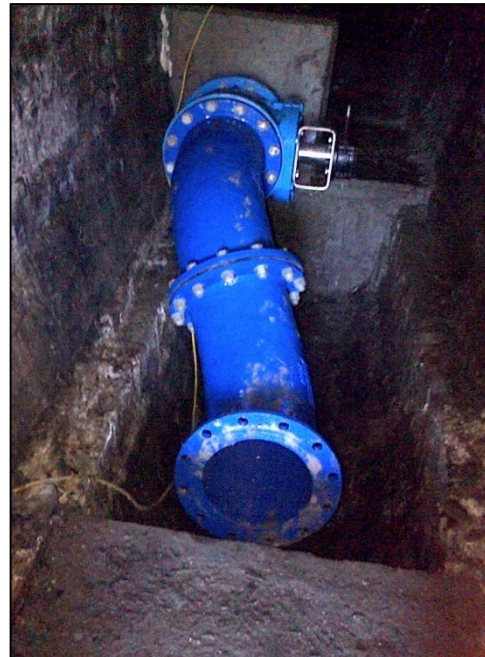
Figure 13. New Drawoff Valve At Downstream Tunnel Entrance
