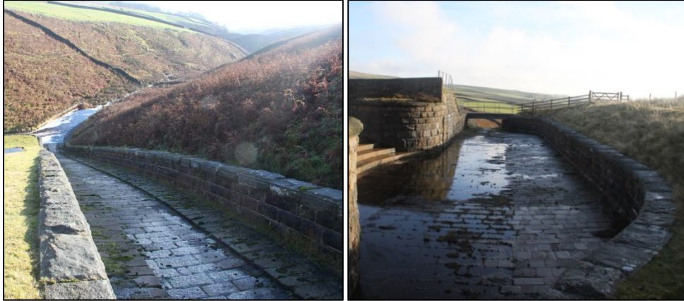
Figure 1. Views of Original Structure
