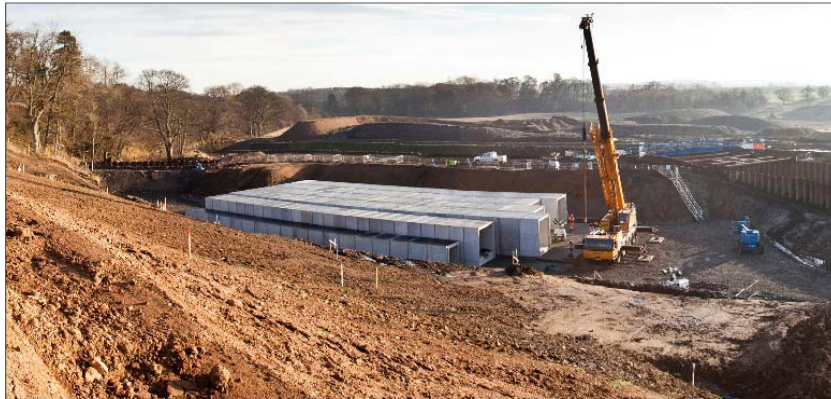
Figure 10. Culvert construction with diversion channel behind
