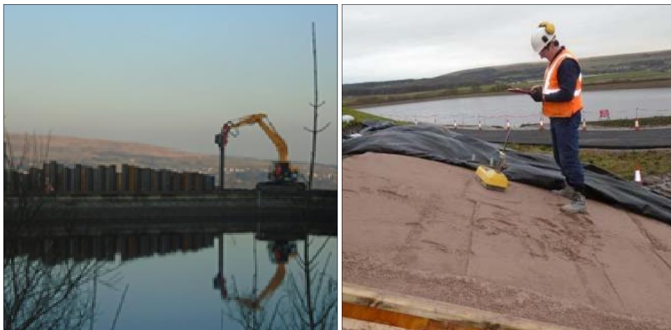
(a) Movax sheet pile installation
