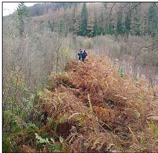
Figure 6. View of crest as found
