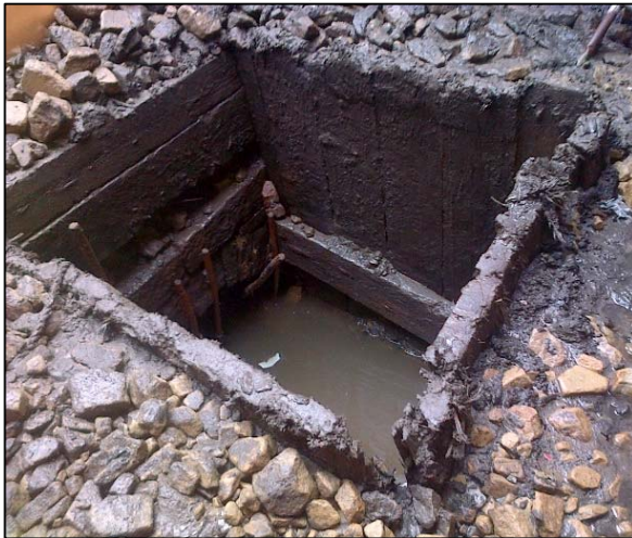
Figure 7. Wooden Hopper on Top of Drawoff Upstream Inlet
