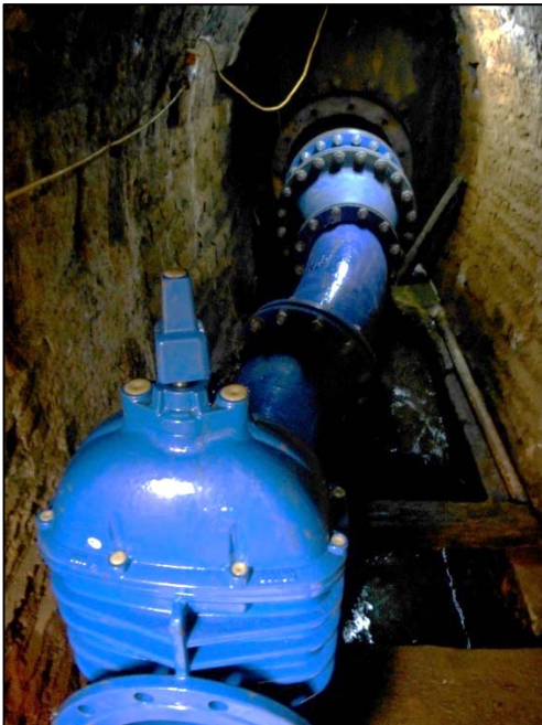
Figure 12. New Guard Valve at Bulkhead
