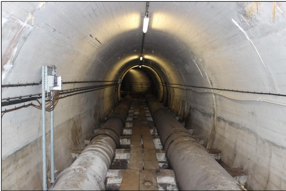
Figure 1. Talybont tunnel looking upstream, with the scour main on the left
