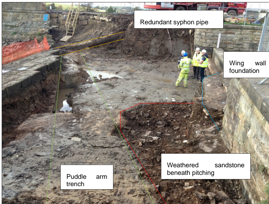
Figure 3: Exposed sandstone, wing wall foundation, puddle arm trench and syphon pipe
