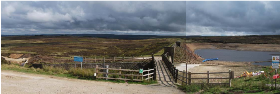
Figure 1: Overview of Keighley Moor reservoir and siphon.
