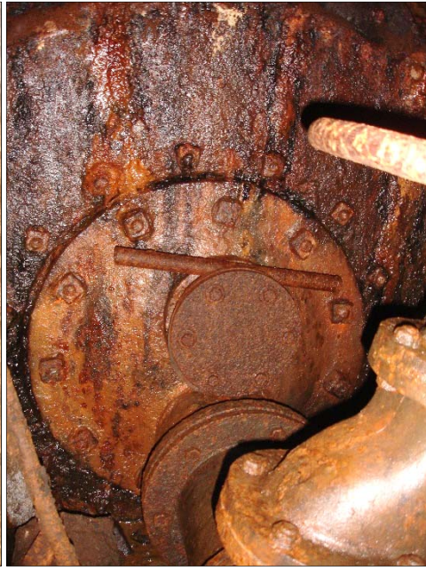
Figure 11. Bulkhead with Railway Pipe Blanked Off
