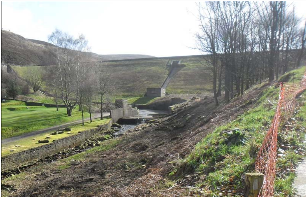
Figure 4. Hurst Reservoir embankment before discontinuance.
