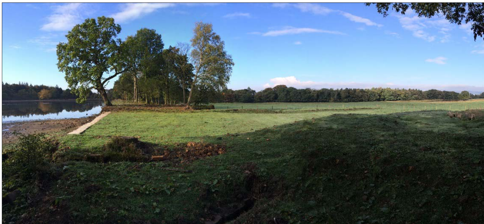
Figure 4 – Swiss Lake auxiliary spillway looking to Mud Pond
