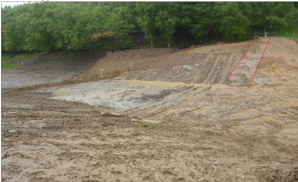
Figure 4. V-notch excavation through Oakdale showing clay core
