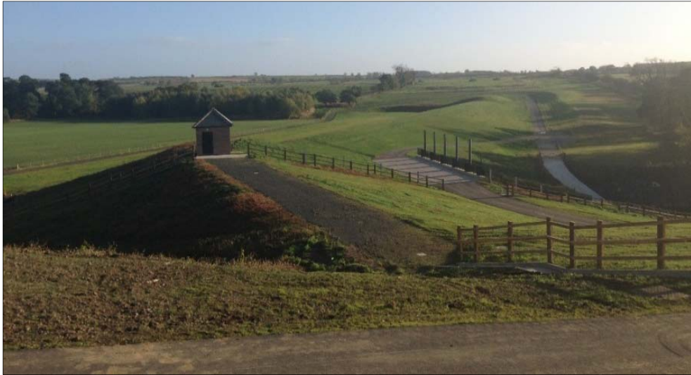
Figure 2. View of Mitford Dam from left abutment
