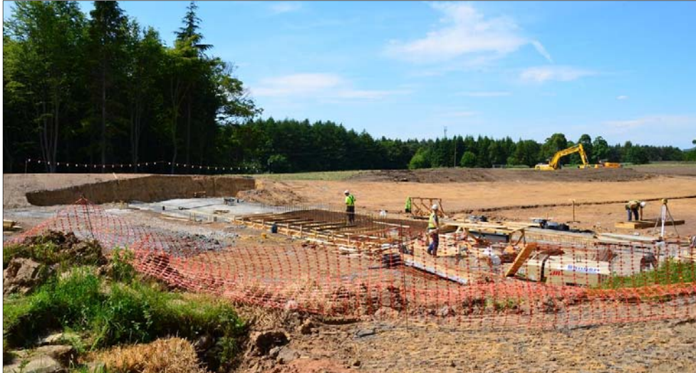
Figure 8 Emperor Lake Weir construction © The Devonshire collection, Chatsworth.
