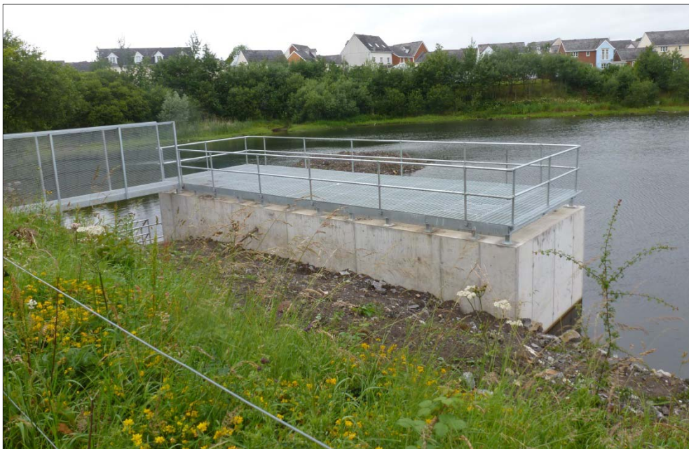
Figure 2. Completed overflow inlet
