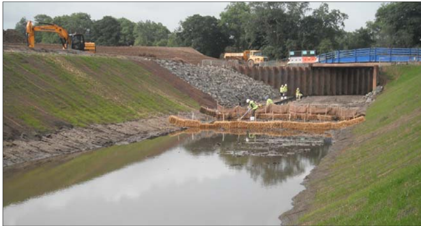
Figure 9. Diversion channel
