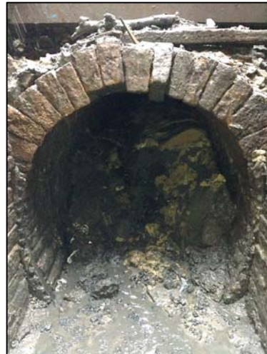
Figure 8. Drawoff Upstream Inlet Culvert Before Cleaning
