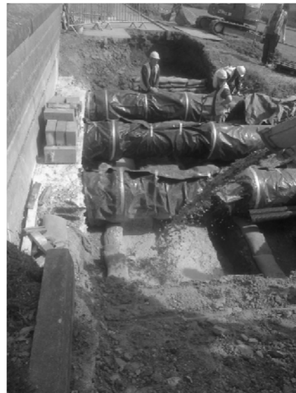
Figure 5: Concrete protection to core during construction of siphons at Pitsford
