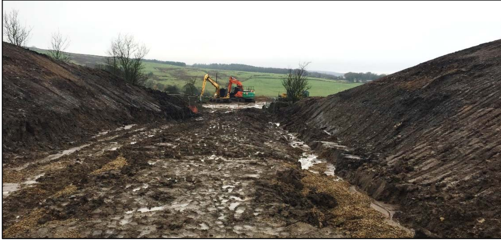
Figure 1. Cutting the notch at Sunnyhurst Hey Reservoir
