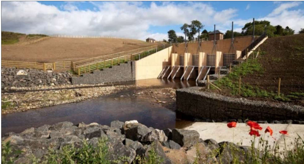
Figure 5. Culvert inlet structure and penstocks
