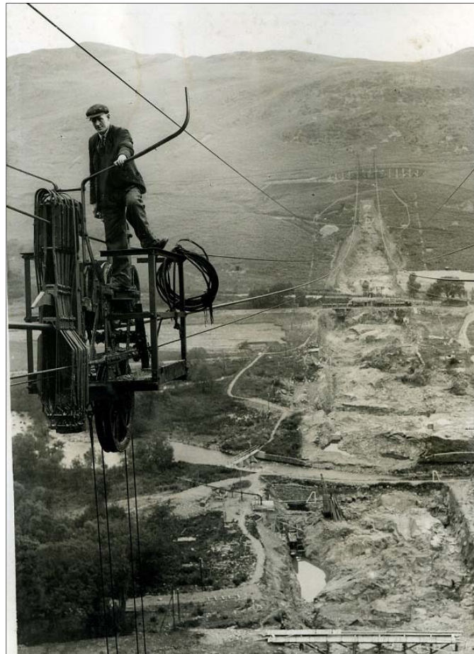
Figure 3: Excavations continue using direct labour
