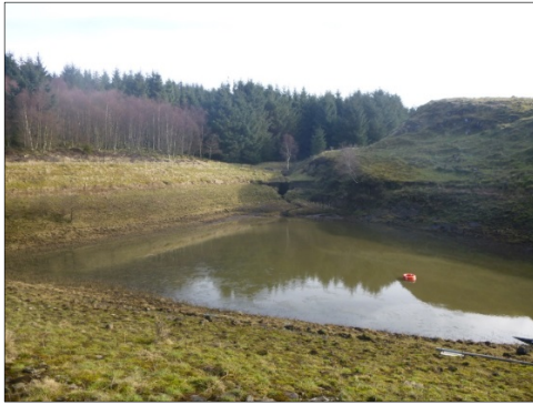
Figure 1: reservoir partially full
