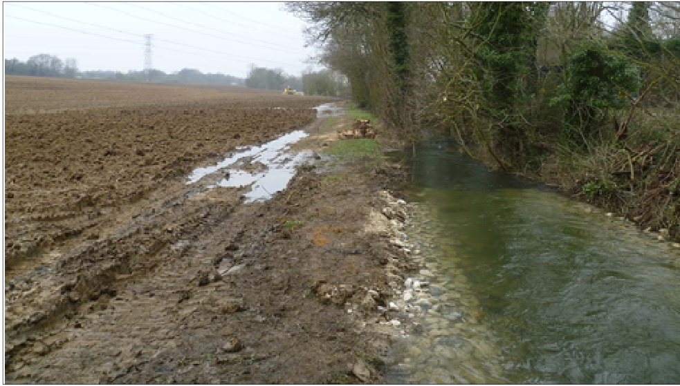
Figure 5. Water spilling out of the watercourse
