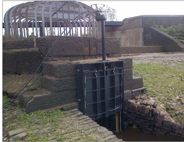
Figure 5. Replacement Penstock
