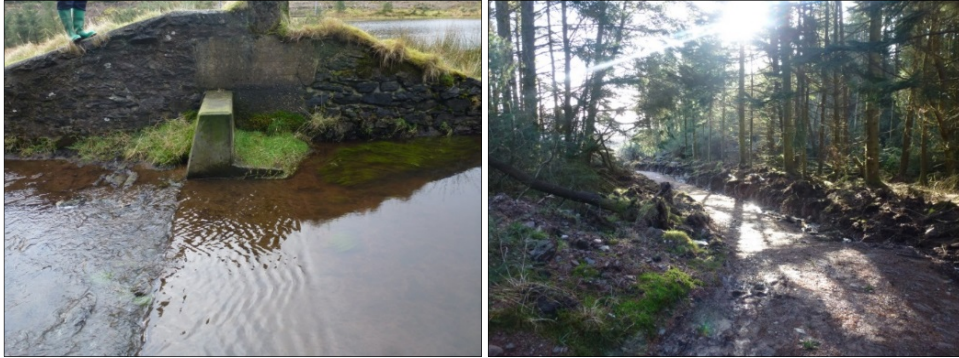
Figure 9: lowered spillway
