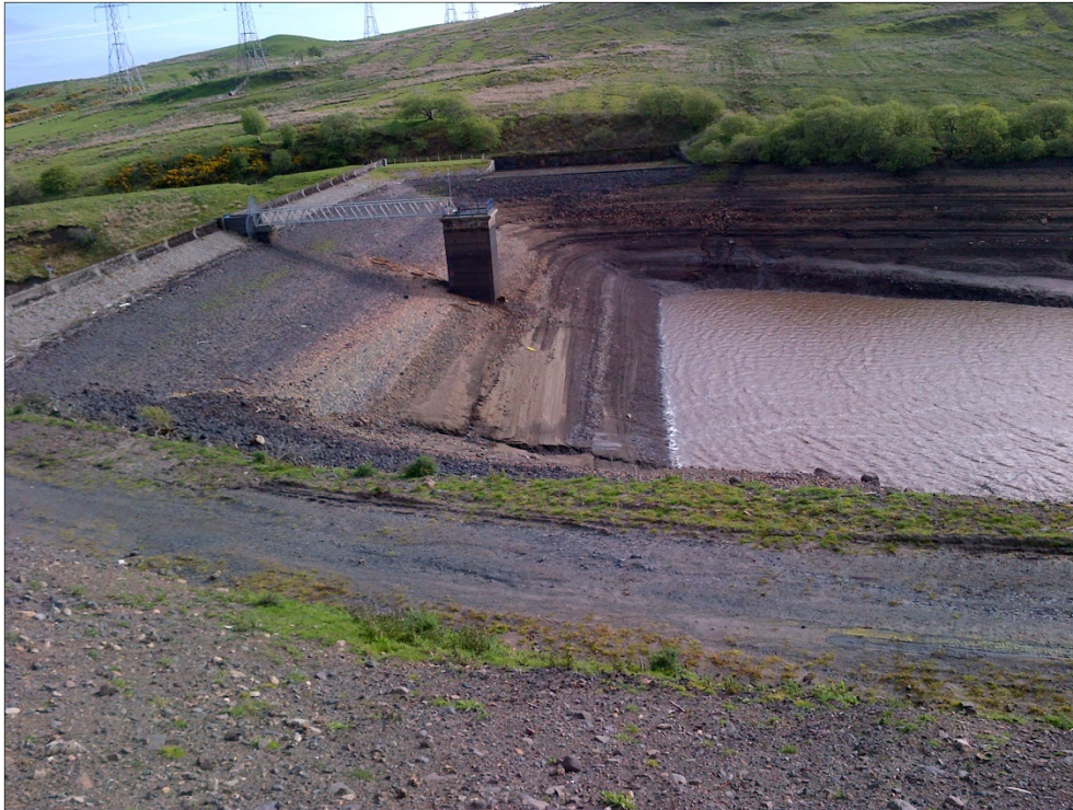
Figure 2. Suspended sediment in a drawn down reservoir from rainfall/runoff over exposed bed.
