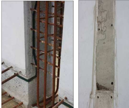
Figure 10. Wall joint detail incorporating hydrophilic strip
