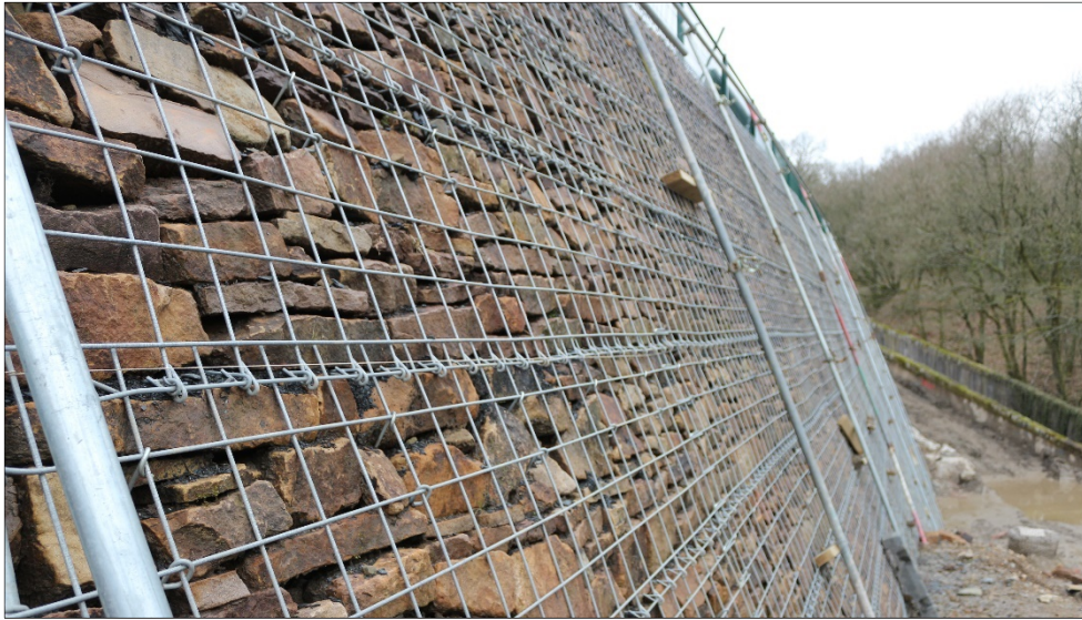
Figure 7 Eco wall nearing completion
