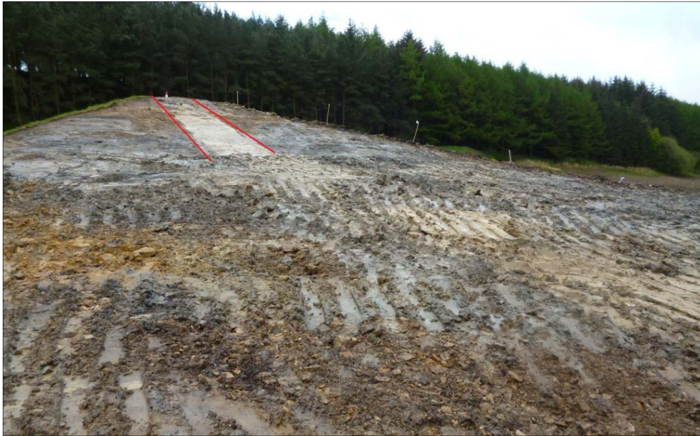
Figure 3. V-notch excavation through Beaver Dyke showing clay core
