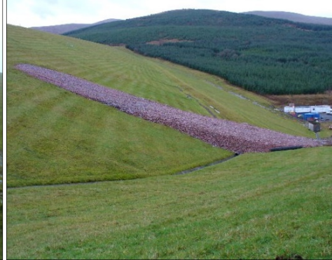
Figure 4. Rockfill berm
