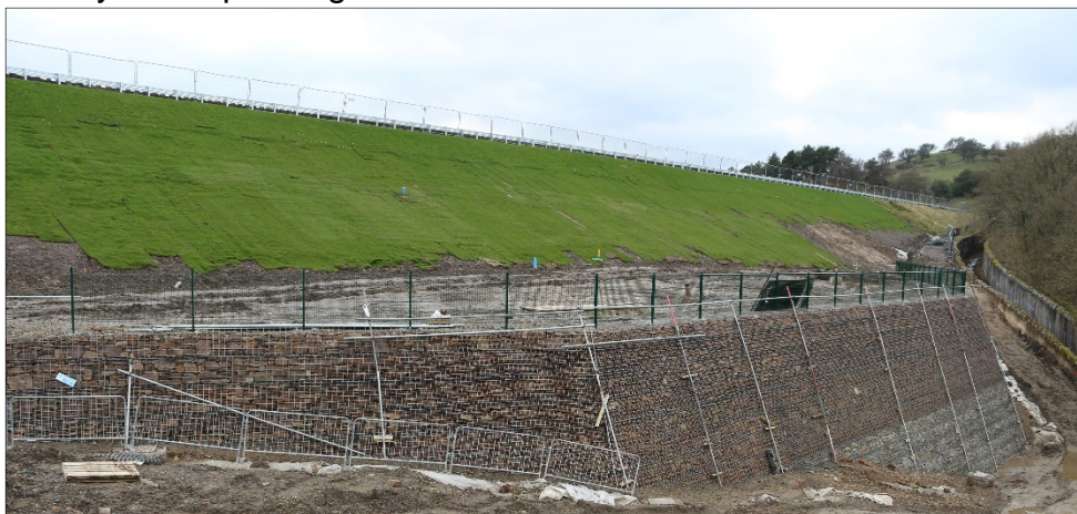
Figure 9. Eco Wall nearing completion
